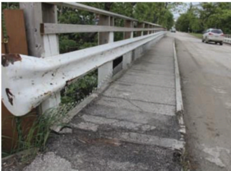
The lack of infrastructure investment compromises the future of rural and northern communities, a new report says. PHOTO: LORRAINE STEVENSON
